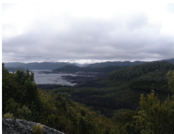
Lake Gordon, Tasmania. Fire damage, 2008 (Jo Wenham)
